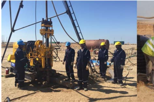
Figure 4: Soil investigation using borehole drill rigs
