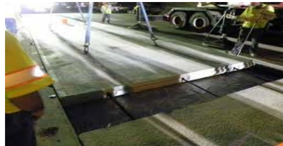
Fig.4 Post-tensioned system
