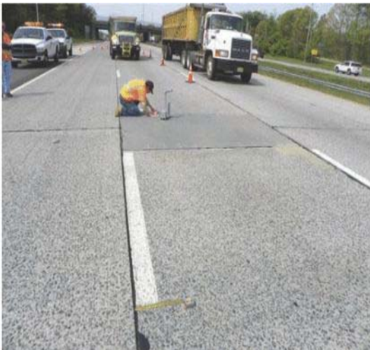
Fig.1 Super slab system in NewYork
