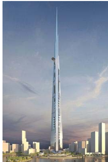
Fig 2 Proposed construction - Jeddah tower
