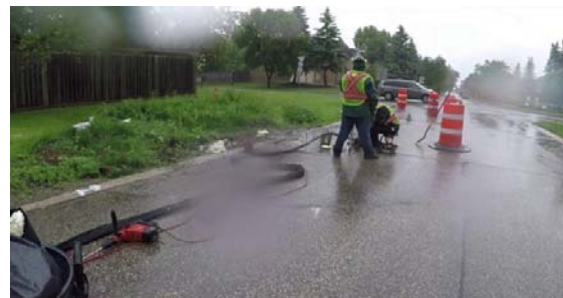
Fig.3 precast slabs under sealed with polyurethane foam
