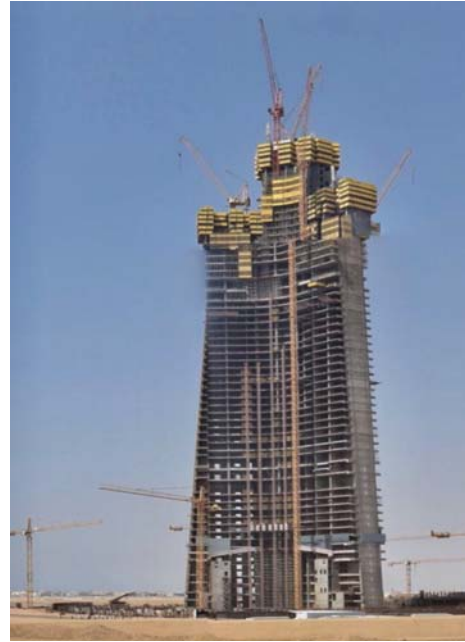
Fig 1 Under construction - Jeddah tower
