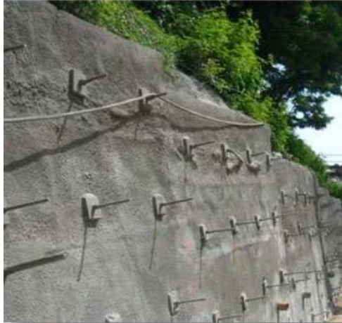
Fig.1.Soil Nailing
